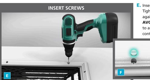
E. Insert each screw working from side to side.
