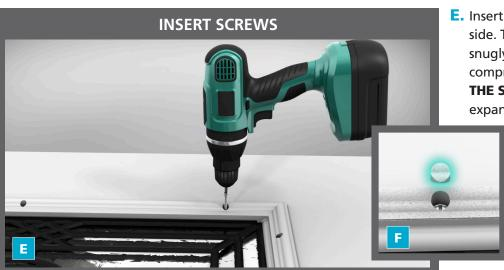
E. Insert each screw working from side to side. Tighten firmly so that the frame fits snugly against the door and the seal is compressed. **AVOID OVER TIGHTENING**THE SCREWS to allow the window to expand and contract. Recommended torque setting around 4 to 6.
